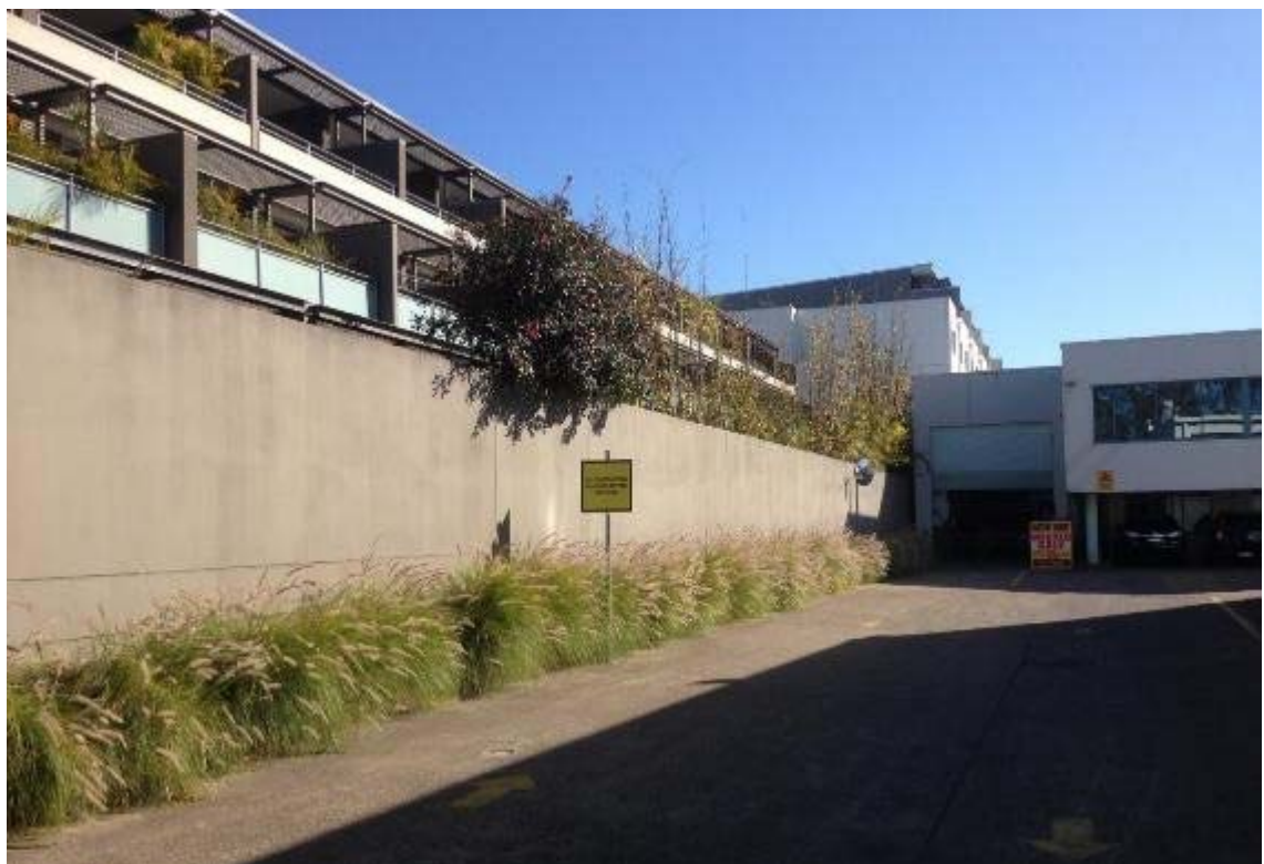
Figure 3: Southern boundary of Site (Nassau Lane dwellings behind wall)
