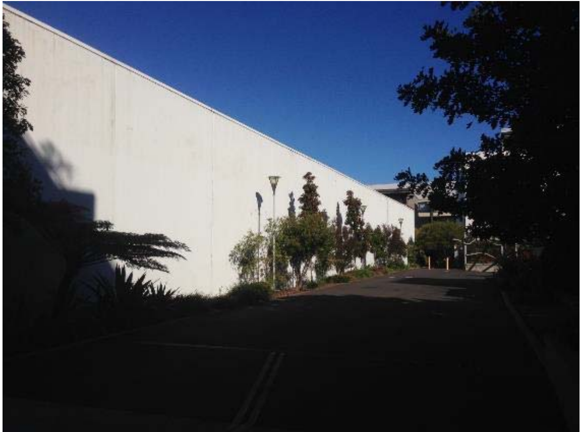
Figure 4: Western boundary wall of Site (adjacent to 'Motto' driveway)
