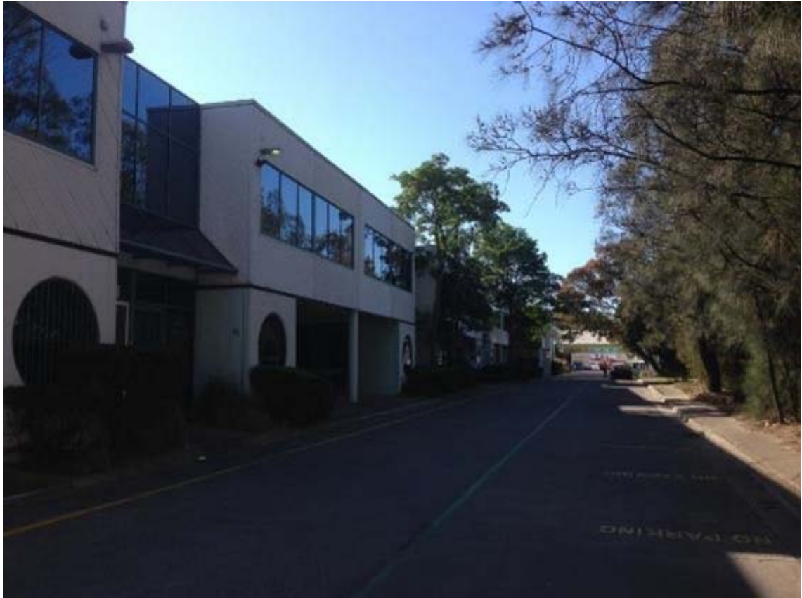
Figure 2: Looking north towards Site from existing driveway
